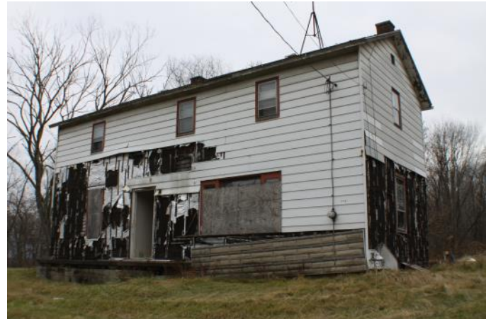
821 Early Rd: DEMOLITION
